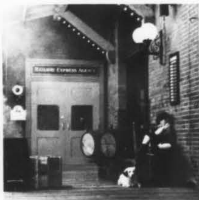
Entrance from loading platform.
