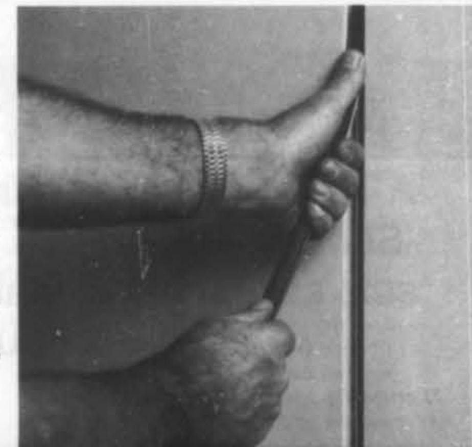
Vinyl strip trims joints providing visual and acoustical seal, permits access to slotted component support.
