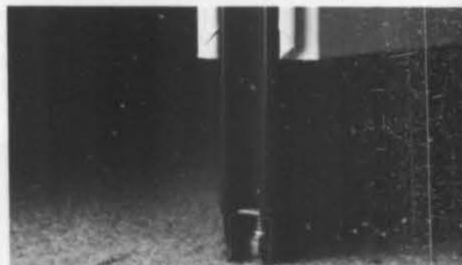
Clip attached to ceiling T-bar forms a "node" to steady top edge support of full-height system.
