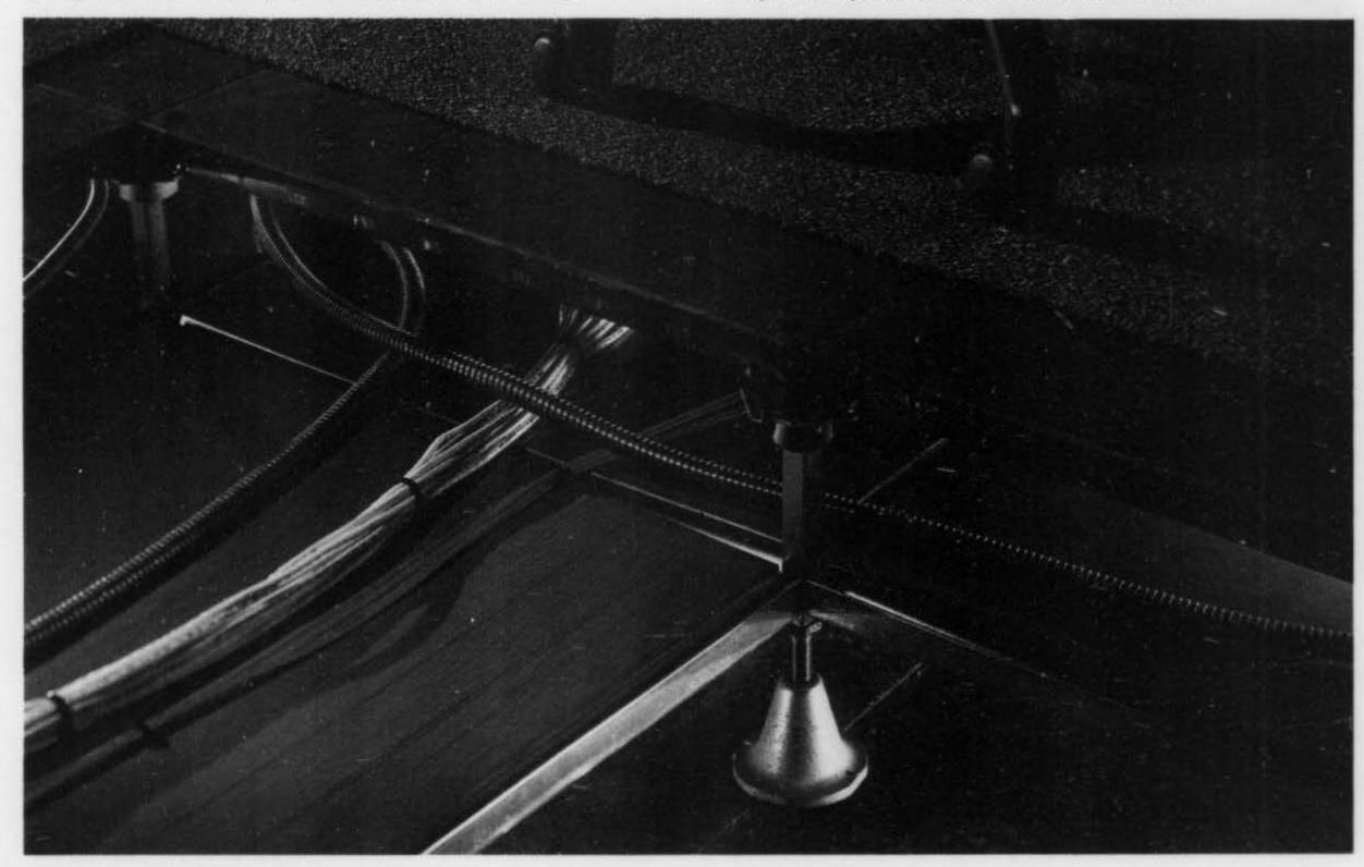
Interface Architectural Resources (InterfaceAR™). Interstitial's™ patented multiple-level raised floor design provides efficient and flexible organization of power, voice, data, and air. Booth 1742. Circle 63.
