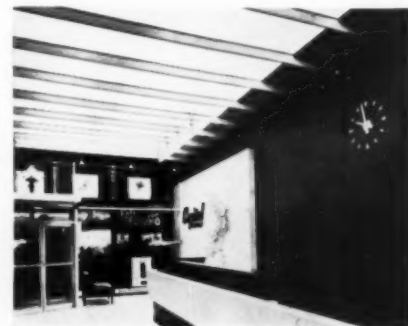
Rolled, corrugated Bakelite vinyl rigid sheet for installation in luminous ceiling. An interior with "Acusti-Luminus" ceiling installed. The projecting ribs are of acoustic material and are sound absorbent.
