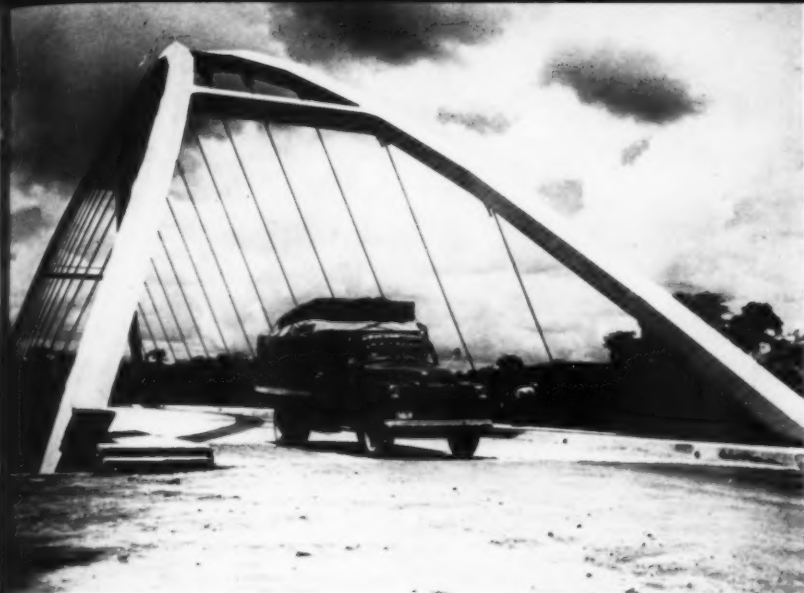
Mexico: Spanning the Rio Blanco near Vera Cruz, this taut-ly strung splayed-arch bridge achieves new freedom with welded steel. By Camilo Piccone, based on a design conception by Dr. Thomas Kavanaugh of New York University.
