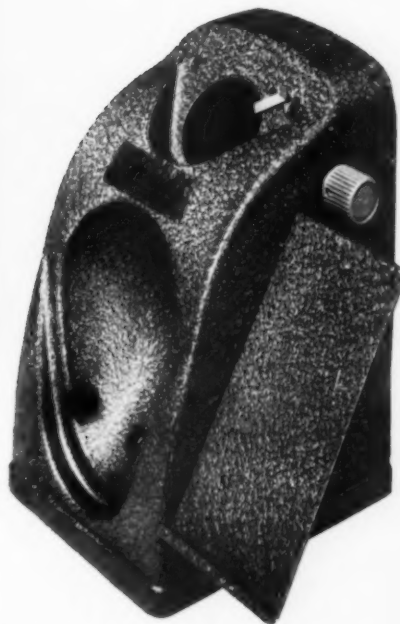
With receiver placed on Fonadek (above), conversation in normal voice may be held without direct contact with instrument.
