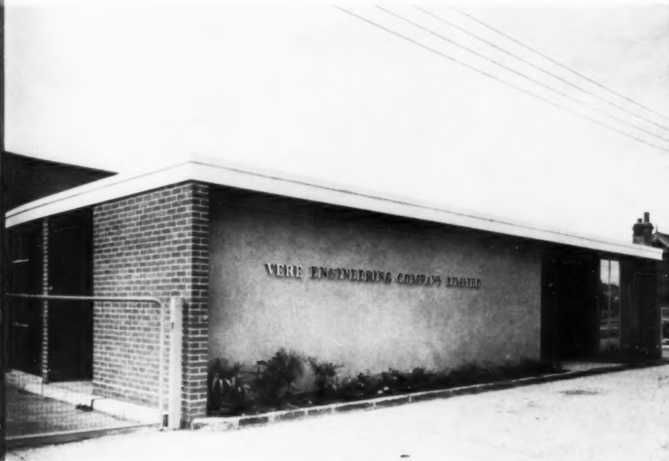
Main facade of Gatehouse from the road.
