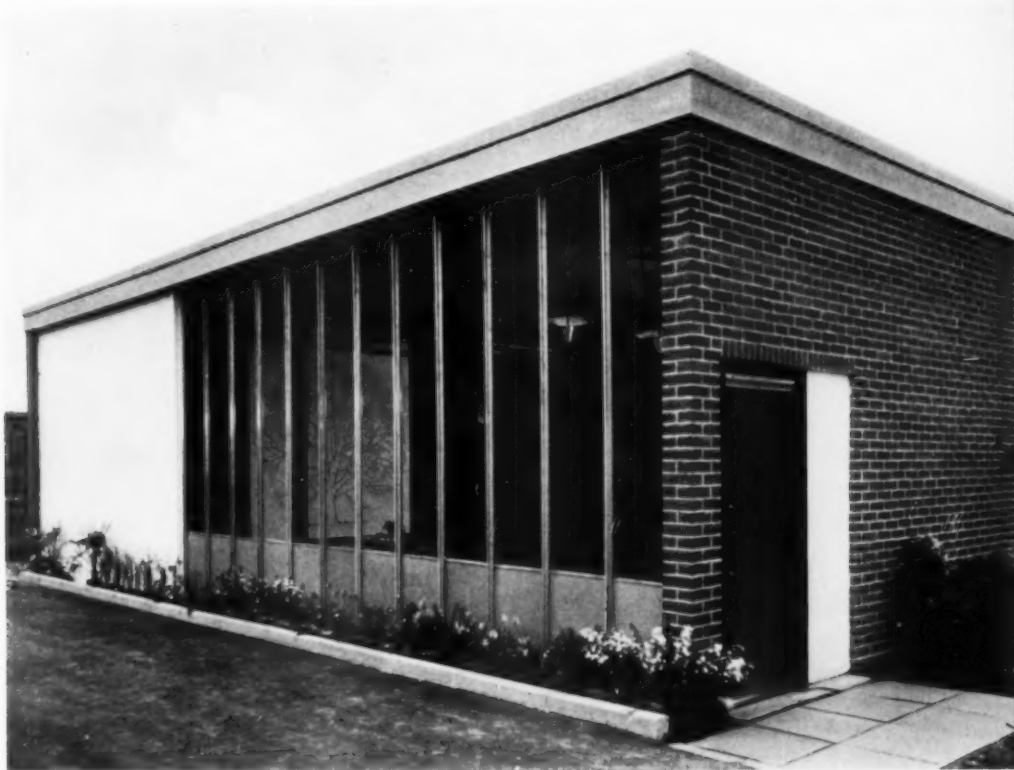
From the outside, the Canteen is a simple brick-ended box tied with aluminum glazing bars.
