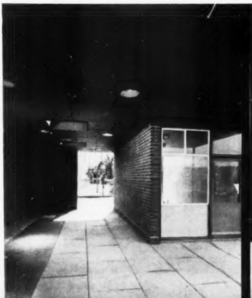
Of combined steel frame and low bearing brick construction, the Gatehouse shelters a policeman, a weighing control officer, and bicycles. Ceiling panels at left are unfaced Bartrev board.
