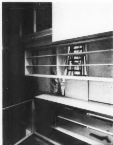
Storage units, under construction, show a variety of board uses.
