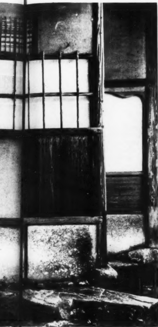
Plaster, often textured with straw, covers wood lath on the walls of old tea houses. Though symbolically rustic, the tea houses show a high order of sophistication in the way the posts are hewn and the walls are proportioned into openings for air, light and people to enter.
