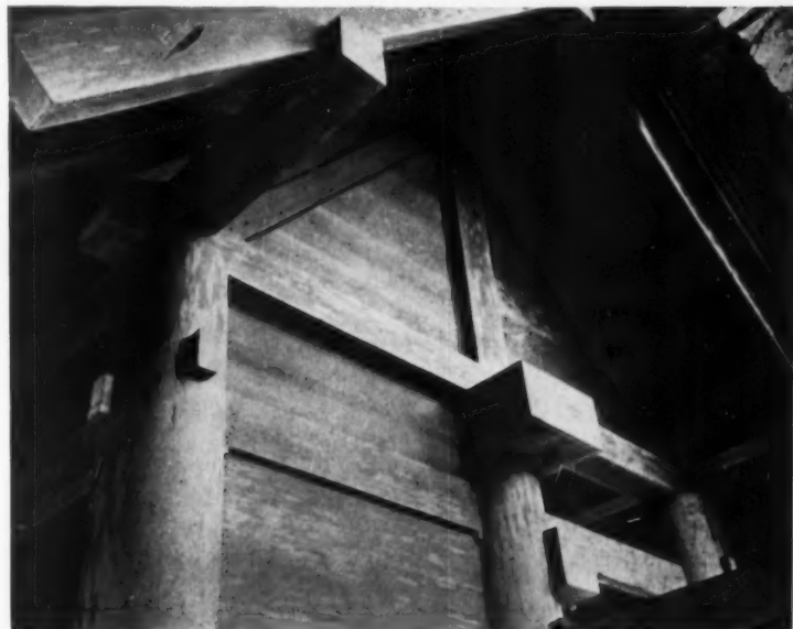
Large wood roofs developed as an expression of the traditional post and beam construction. In ancient Buddhist temples (left) a complex system of rafters and brackets was needed to hold them up—to compensate for the fact that they were not based on the logical truss system of their Chinese prototypes. It is paradoxical to find such an elaborate effort to maintain an illogical convention in the Buddhist temples, while the Shinto shrine of Ise (above) shows an absolute respect for the organic use of materials. Though it is one of the earliest examples, it is perhaps the ultimate expression of the beauty which comes from total eliminations of the insignificant.
