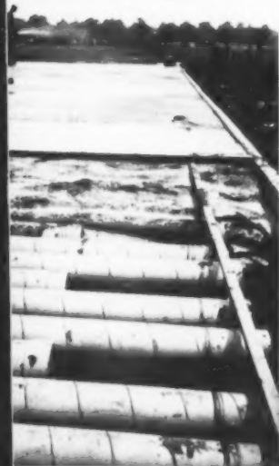
Sonotubes, prefabricated forms for pouring concrete posts are kraft paper and chipboard, polyethylene-coated inside; Sonovoid tubes save material and weight by becoming part of the poured concrete slab (left). Sonoco Products, Hartsville, S. C.
