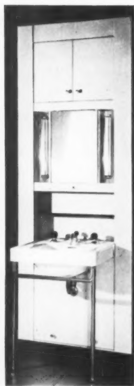
Left: An early "modern" lavatory designed by George Sakier was part of a prefab panel that fitted between studs. It wasn't popular with plumbers.
