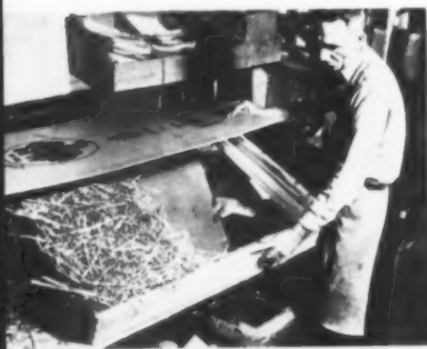
Continental Can's Payoffpak for wire is designed as a 3-in-1 labor saver: a fiber winding drum for wire off the drawing machine, a shipping carton and later a dispenser.
