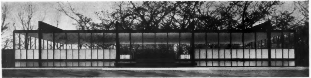
Mies van der Rohe's newest addition to the I.I.T. campus, in model.
