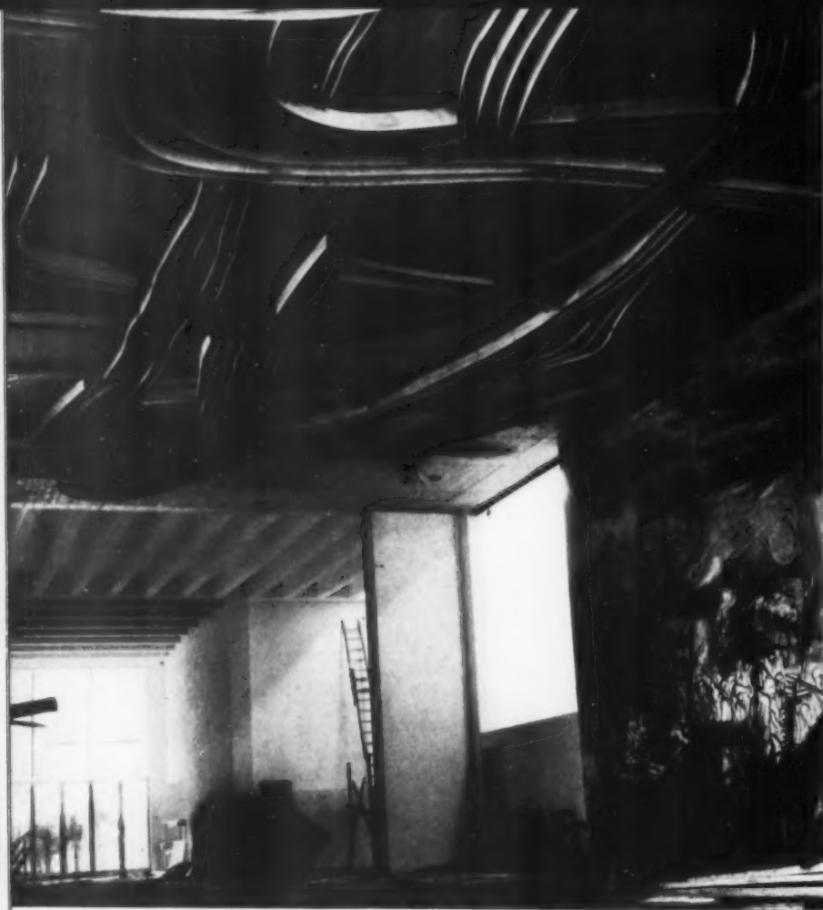
Ceiling of curved plywood strips in entrance hall to Palazzo dell'Arte.
