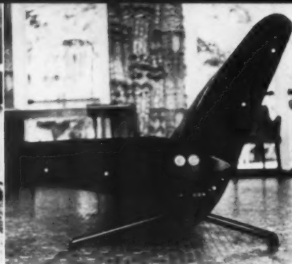
A sofa bed used throughout the Palazzo has an underside knob which adjusts the angle of two foam rubber wings. Borsani.
