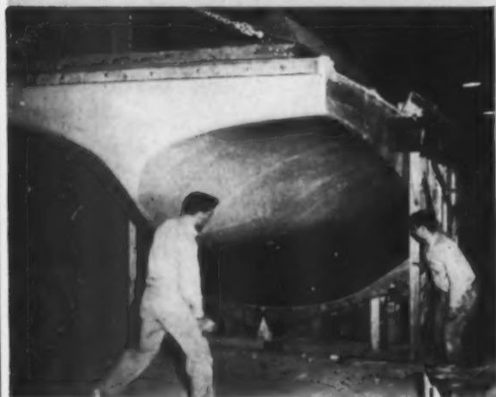
Preparing after section for • assembling with hopper section.
