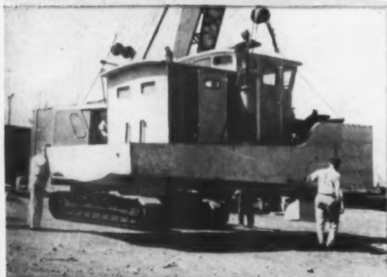
• Removing forward section from mold.
