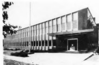
Blue and gold aluminum panels sheathe Alcoa's Cincinnati office, one color per wall.
