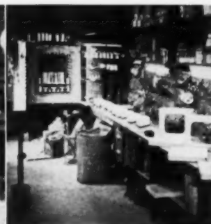
Trude scrapes mold marks from dry pieces, now white. Harold dips each piece in glaze for final finish before putting it in kiln where heat fuses clay into hard white porcelain. Firing cycle takes one day to heat slowly, two more to cool off again.
