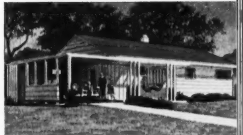
Leading manufacturers of prefabricated homes use Presdwood for siding, gables, doors and walls.
