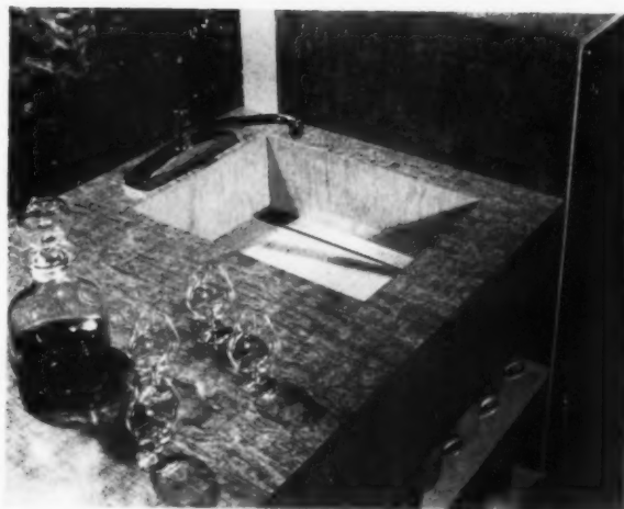
This sink counter (Anshen), and all non-copper surfaces in the kitchen units, are finished in two shades of high-density resin-overlaid plywood, which is hard and glass-smooth.
