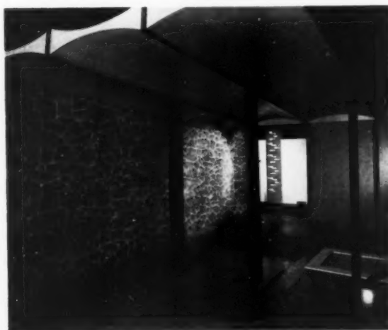
Stressed-skin plywood columns (Anshen) support roof.
