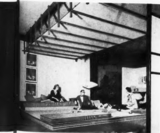
The conversation platform ( \frac{3}{4} " plywood 6" off the floor) by Choate replaces a furniture group, keeps seating, circulation apart.
