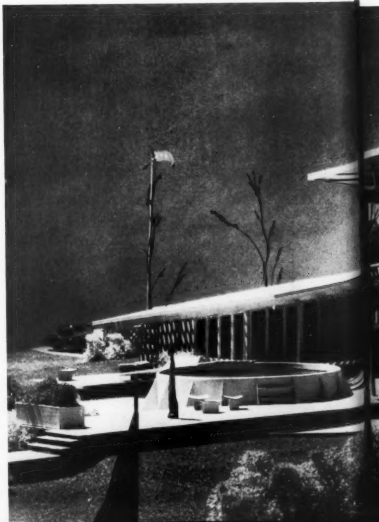
Stressed-skin plywood columns (Anshen) support roof.
