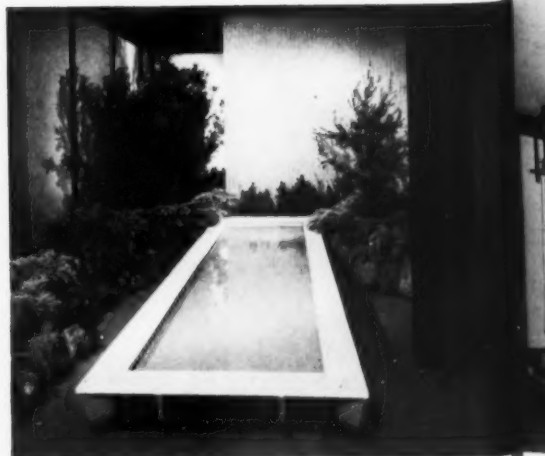
This garden reflecting pool (Anshen), all plywood with a bottom of 3' x 12' panels over a web, can be lighted from beneath.
