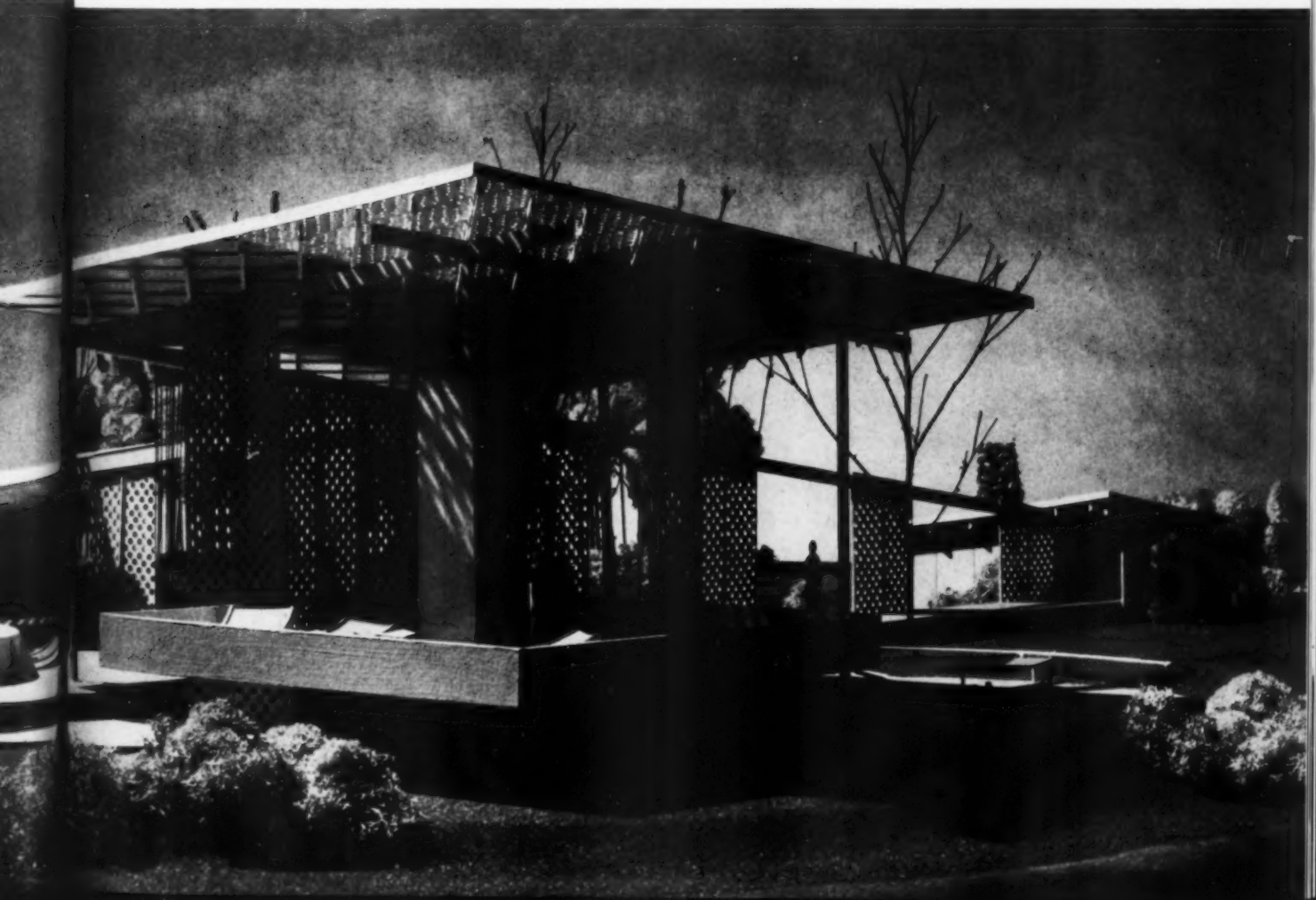
Trademarkings on Plyscord wall and roof sheathing (through arch) can be used as nailing guide. One use shown for molded angles. Plywood leisure house has three units: a windowless fireplace structure (right), a sun-shelf and arbor (middle), and a functional center.
