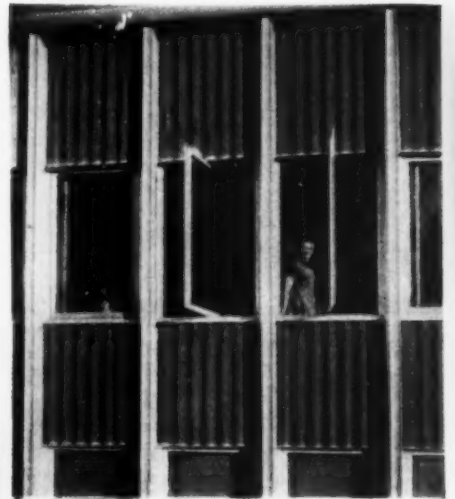
↑ Color-anodized curtain wall panels
