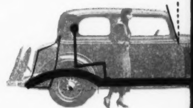
1933 — Buick. The first built-in trunk makes the trunk extend beyond the back wheels. The front end remains boxy. The windshield is slanted slightly and the fenders are more rounded. A definite frame kick-up over the rear wheels — on most models by this time — lowered the car, giving a more aerodynamic body lines. The wheelbase on this model is 127 inches.
