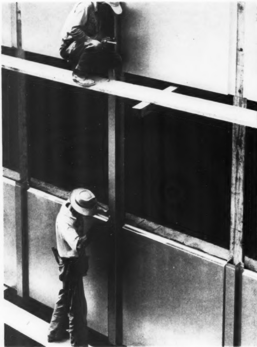
↑ Color-anodized curtain wall panels
