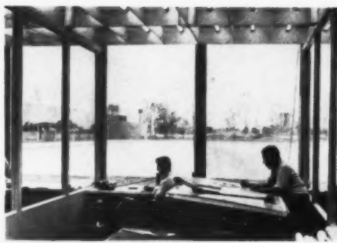
Curtain walls of glass and porcelain are set in aluminum frames by a new method, developed by GM and the architects, using a neoprene gasket like the one that holds auto windshields in place. Modular system permits great control of daylight: full usage, as in the Process Development building above and the Engineering building at the left, or controlled usage, as in the Dynamometer building below.
