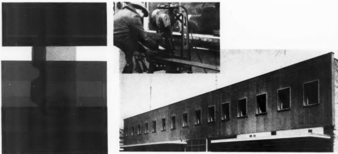
Porcelainized aluminum panels may be sized in the field (above) and will not erode at the cut edge. They can revitalize the facing of an old building (below) by providing solid blocks of durable color.
