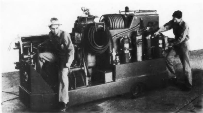
115 In-plant fire truck Ansul Chemical Co., Marinette, Wis. St. Clair Industries, Detroit, designers and manufacturers
