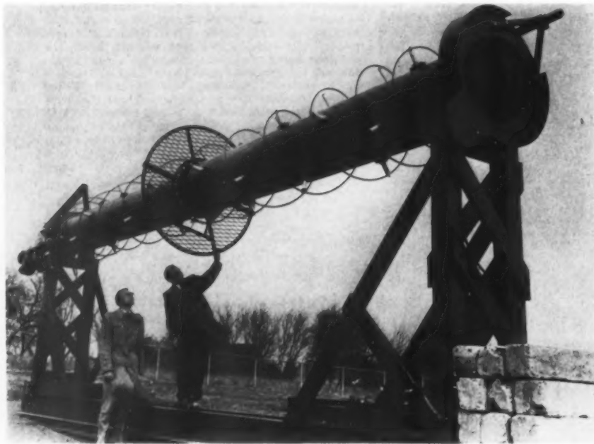
New General Electric "high-channel" television transmitting antenna.
