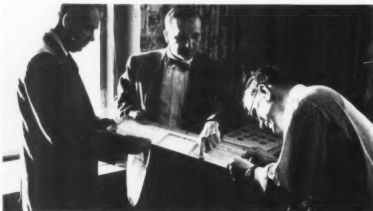
Weeks later, Kohlmann and Oles return to Boldt's office with a prototype panel molded by GATX in fiber-glass reinforced polyester. With Wojtowicz, they check it for accuracy and, after approval, give GATX the go-ahead for production molding.
