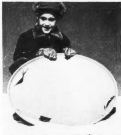
↑ Kalamazoo Sled Company gives a new shape to an old sport. Useful in deterring youngsters who like to coast on the best family tray, this lightweight "Flying Disc" is molded from G-E polyester resins and fiberglass.
