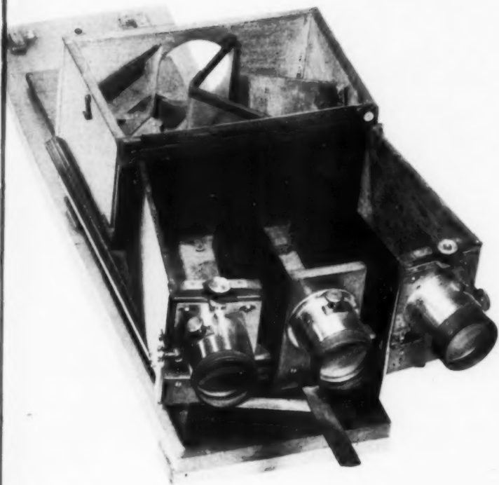
The "Kromskop" of 1892, first color projector; used three black-and-white negatives and three color filters, red, green, and blue; light source—electric arc lamp inserted at back.
