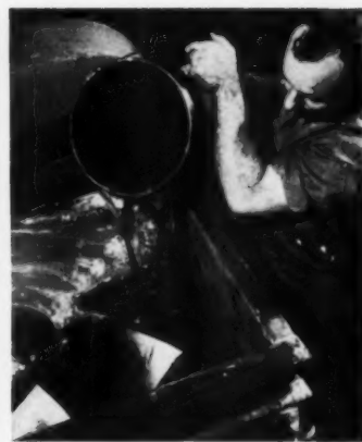
Glass fibers, clay filler, mold lubricant, black pigment and benzoyl peroxide paste pigment are typical ingredients for premix molding. Beaker contains vinyltoluene type polyester resin, being poured (right) into mixer.
