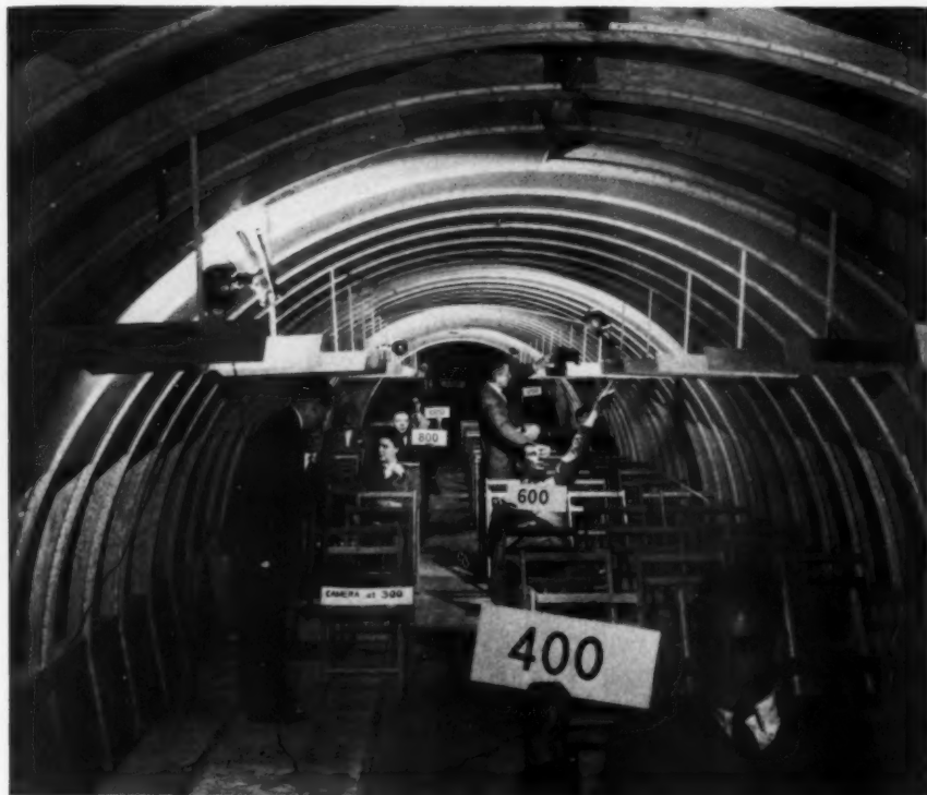
The passenger service unit is adjustable to the seat spacing, goes under the hat rack.
