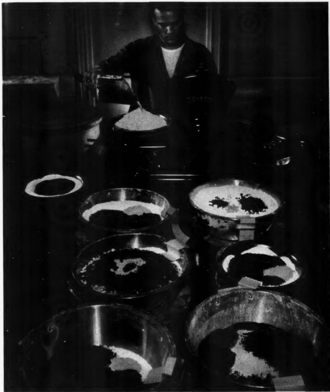
Pigments are mixed for full-scale production of Barrett's Plaskon molding compounds.
