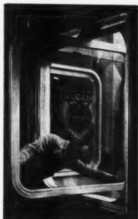
Fitted with inflatable rubber tubing for weather protection, Alcoa Building windows pivot a full 360° for cleaning.
