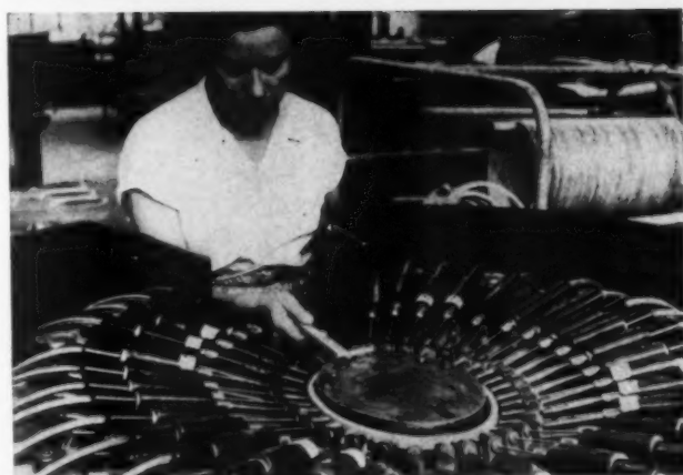
Thirty-two holes are drilled simultaneously in a racket frame.
