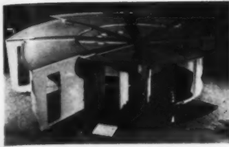
French all-plastic house (L.) has round core of polyester ribs and sections; 3 bedrooms may be added as modules.
