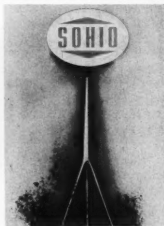
(→) Sign standard of tapered tubes
