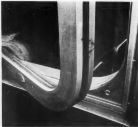
Fitted with inflatable rubber tubing for weather protection, Alcoa Building windows pivot a full 360° for cleaning.
