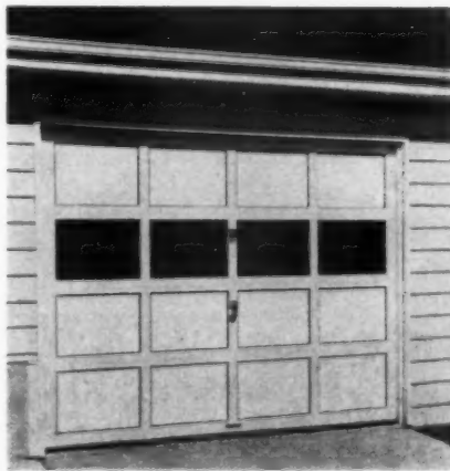
Shadowvent siding, made of Presdwood lengths, "floats" on a crimped aluminum strip nailed to the building; every 8 inches is a vent to reduce moisture build-up. Left, the garage door of tempered Masonite board; below, Tracy Kitchen cabinets.
