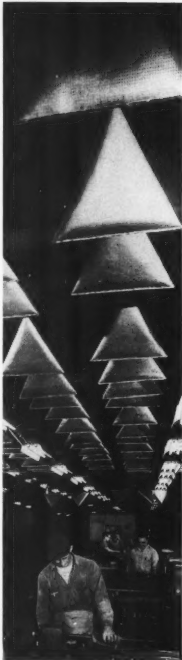
Left, "Acoustosorber" units, pyramid-shaped, are suspended from factory ceiling. Two inches thick, they are perforated aluminum foil with mineral fiber blanket. Below, Kepes-designed "Fantasia" for acoustical tile; "Festoon" design for expanded metal mesh.
