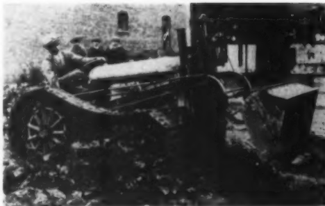
Original shovel attachment, mounted on Fordson tractor in 1922, was called North Hydraulic Digger.
