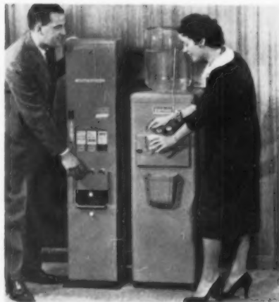
↑ Mosler Safe Company displayed their new Day and Night Deposit, a redesign by Henry Dreyfuss. The surface of the safe is brushed, corrosion-resistant stainless steel.
