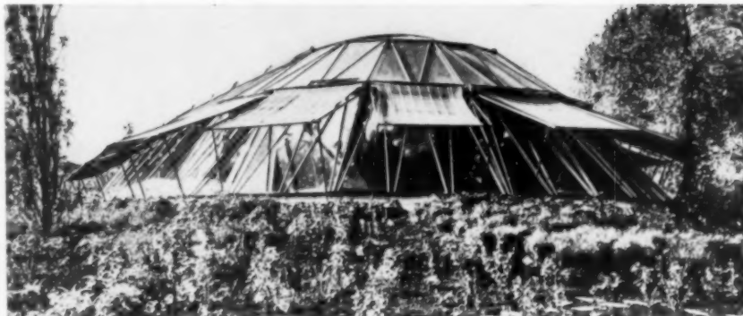
1. Plant exhibition house by Bernhard Hermkes adds tent-like flaps to glazed dome
