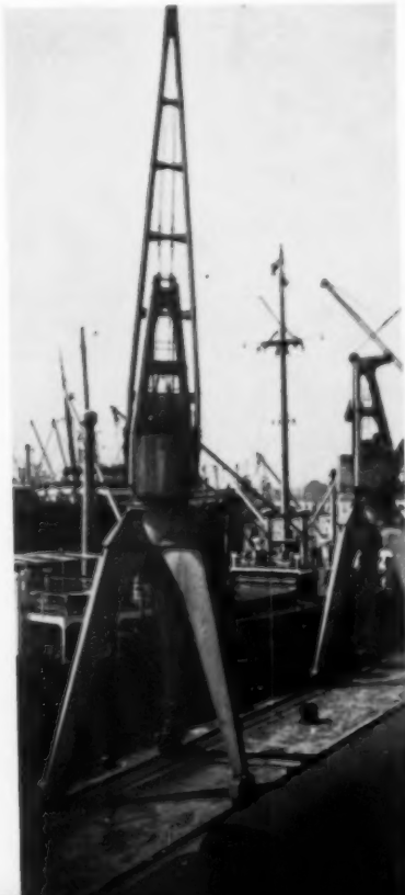
Cranes take different forms but employ new principle shown in diagram: center-post supports slewable section, moves with it. Roller bearings at top and bottom of post absorb vertical and horizontal forces respectively. Counter-weight is now placed in legs; either three (left) or four (above) legs are used.
