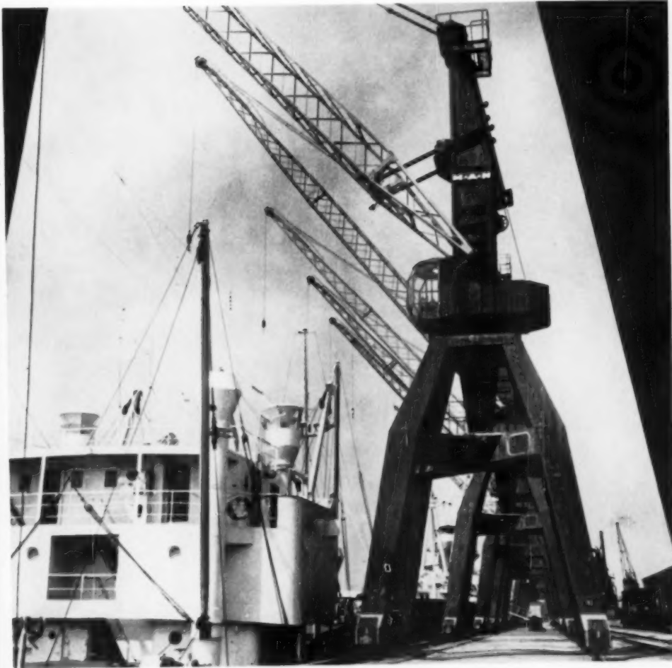
Cranes take different forms but employ new principle shown in diagram: center-post supports slewable section, moves with it. Roller bearings at top and bottom of post absorb vertical and horizontal forces respectively. Counter-weight is now placed in legs; either three (left) or four (above) legs are used.
