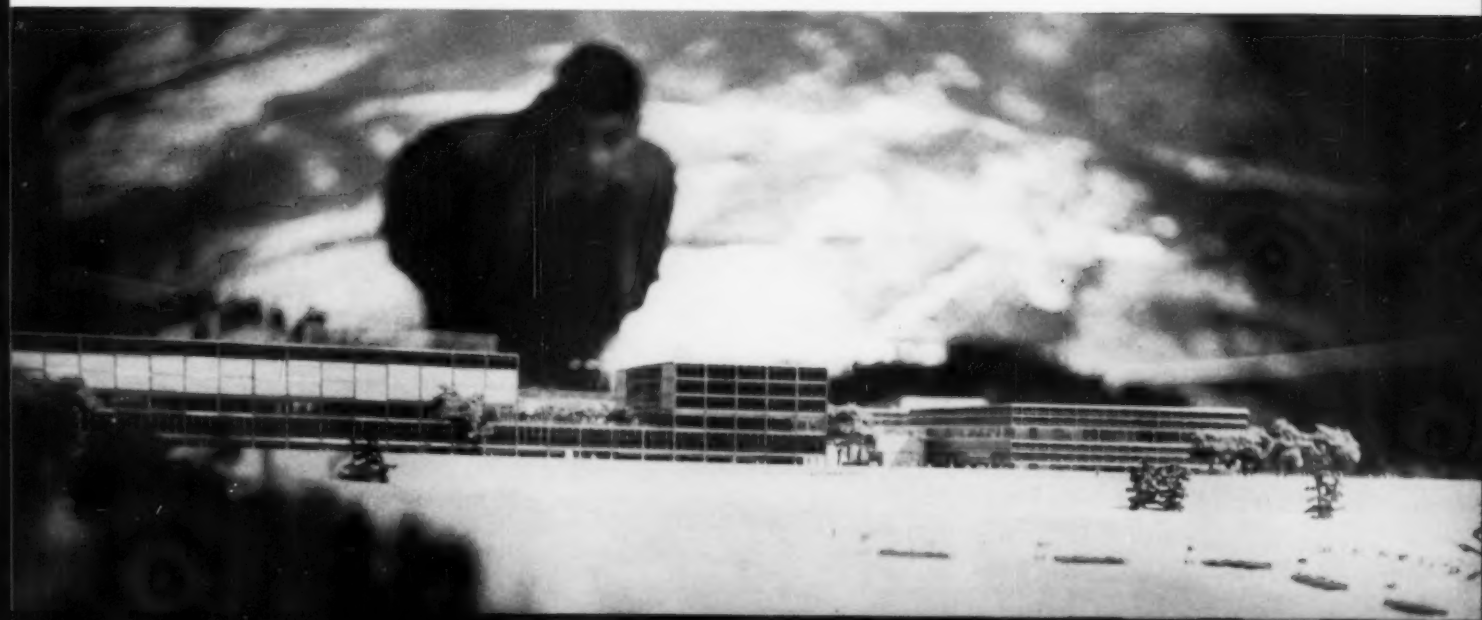
Not without receiving a few brickbats from Congressmen, the Air Force Academy design by Skidmore, Owings and Merrill escaped with its glass walls and contemporary character. Occupying about 400 acres, seven major buildings will be erected on paved platforms, in a unified scheme to provide cadet living quarters centrally, and administration, social, dining and academic in other halls.
