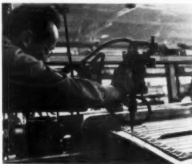
Large structures joined by Budd's "shot welding" process
