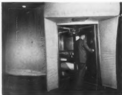
Air-pressure alone supports the Airhouse
