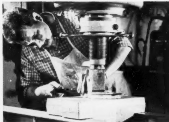
Trim parts, made of stainless steel in production, are machined from brass, and chrome-plated for prototype model.
