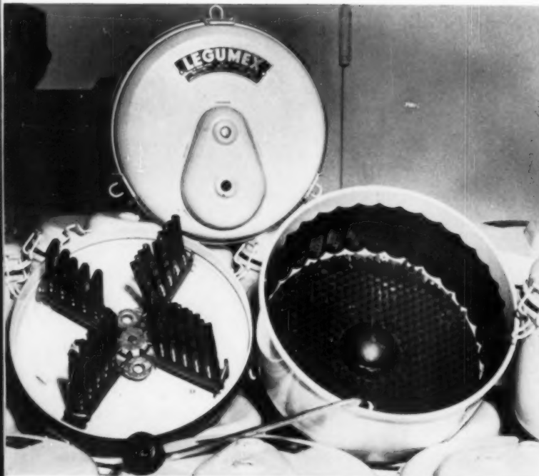
A peeler that can cope with a potful of vegetables, the Legumex has flexible peeling fingers in an inside lid (top right). As the handle is turned the vegetables are gently scraped by the rotating peelers, the abrasive sides and bottom.
