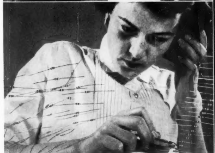
Final check of diode with special orientor (at Hughes Aircraft).
