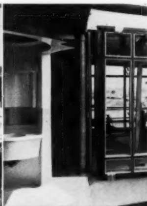
Framing system, right, for the eight window walls is made of laminated wood.
