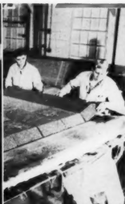
Urethane insulation being foamed-in-place for a modular section.
