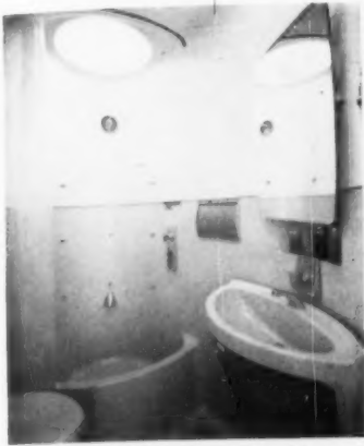
† Children's bath contains shower and adjustable sink. Clothes washer-dryer is recessed in the wall.
