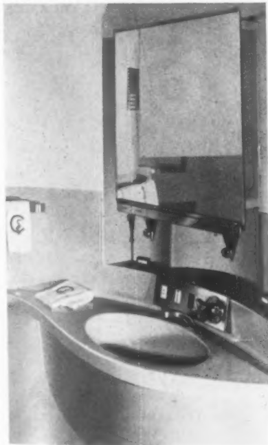
† Medicine cabinet which has been recessed in wall has fluorescent lights attached. Below it is a holder for electric toothbrushes, shaving cream, soap. Line of lavatory flows in with line of the wall.
