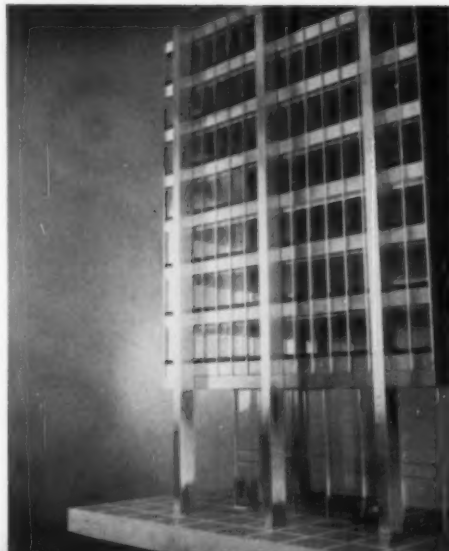
First model expression of new Chase Manhattan Bank building (white block above) and surrounding downtown Manhattan area, was followed by sectional model of base and lower floors (right) to determine fenestration and other details. Ted Conrad (in center, right above) carried through project in Jersey City shop.
