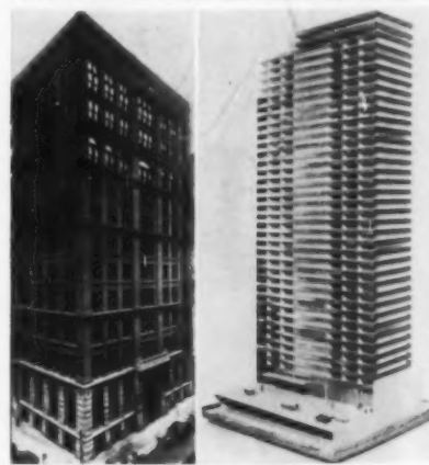
Recap of curtain wall history: first one by Jenny (l.), latest and tallest (r.).
