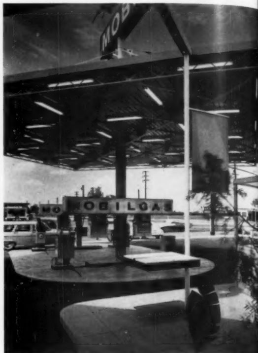
Gas station by architects Smith & Williams (The Roulac Co., research and construction), for General Petroleum Corp., simplifies shelter to metal roofing.
