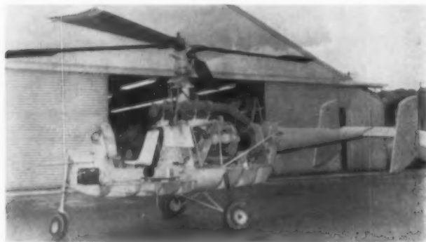
A pressure jet engine drives the Monte-Copter Model 10A.
