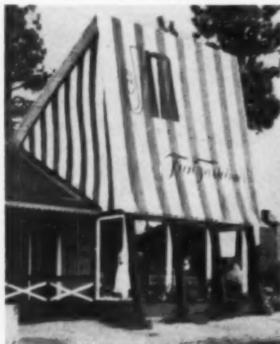
Resort fashions store at Lake Tahoe by Walter Landor Associates for Joseph Magnin Stores: canvas roof and sides can be packed away to duck winter snowstorms.
