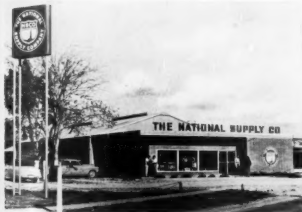
Prototype supply shed, designed by Dreyfuss, is adapted to field conditions throughout the country.
