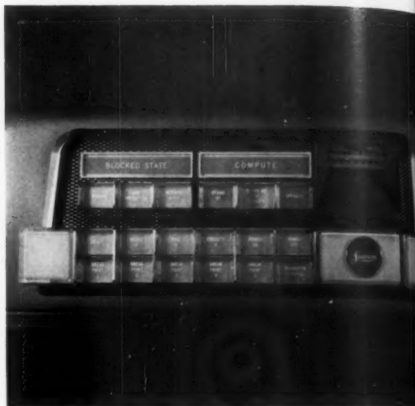
Panel of Librascope's LGP-30 computer helps simplify its operation.
