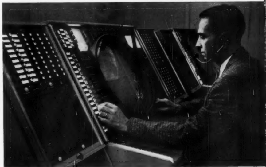
Prototypes of console manufactured on a pilot line production run—an aid for full scale production study—were used in SAGE computer trial operations.
