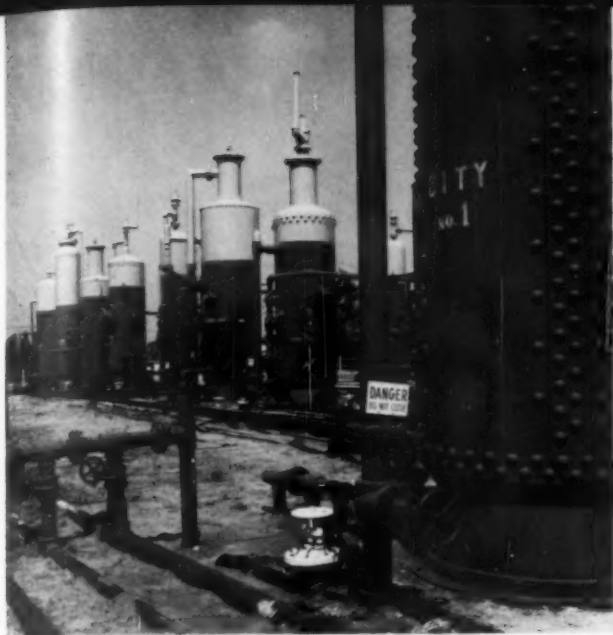
Uniform color bands neaten irregular oilfield equipment.
