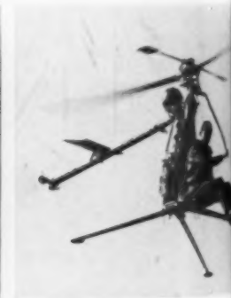
242 One-man helicopter Hiller Helicopters, Palo Alto XROE-1 Rotorcycle, built for Navy. Folding and portable, only 270 lbs., it may be assembled and flown in few minutes.
