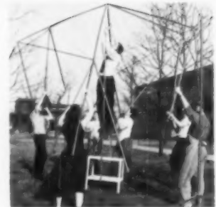
Raising loosely strung structure proved a problem. Center post was added temporarily, dome lifted like umbrella.
