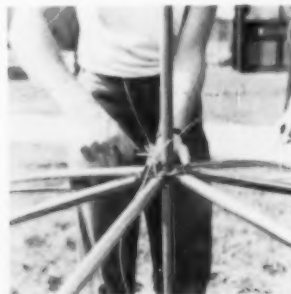
Raising loosely strung structure proved a problem. Center post was added temporarily, dome lifted like umbrella.
