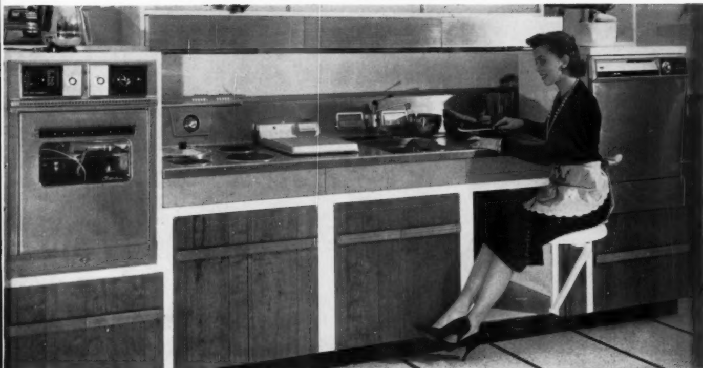
Eleven-foot modular kitchen has many improvements in detail and arrangement over first production model introduced in 1956: oven and dishwasher are set on wood cabinets to put them at more convenient height (both are standards of 1958 line); seven-foot counter top has two-level sink, sliding maple cutting board, four burners; swing-out stool lets the housewife sit at her tasks. Light is provided by three overhead drawers which automatically turn lights on when pulled out. One includes a ventilating hood.
