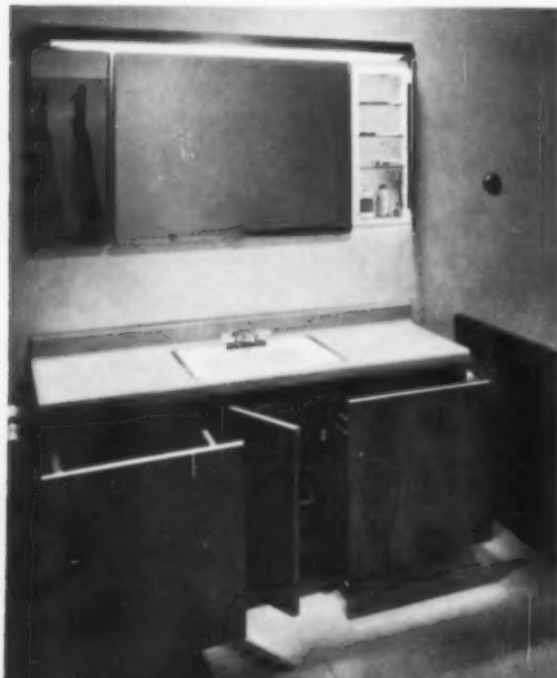
Valet unit has pull-out laundry hamper, medicine cabinet, towel racks for each cadet, plus section for shoe-shine equipment. Perforated bottoms provide ventilation. Rifles (reflected in mirror) will not be issued.
