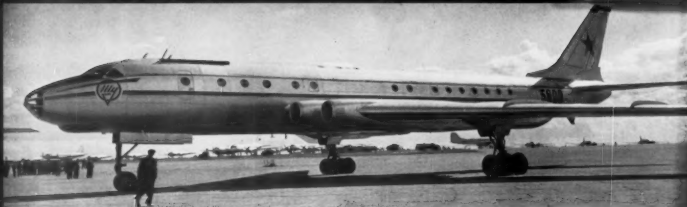
The powerful TU-110 has four turbojet engines, cruises at a speed of more than 620 miles an hour, and carries about 100 passengers. This ship, like the TU-104 which won him a Lenin Prize recently, was designed by the well-known Andrei Tupolev.
