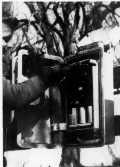
Plug-in transistorized units at rural terminals have increased phone service.
