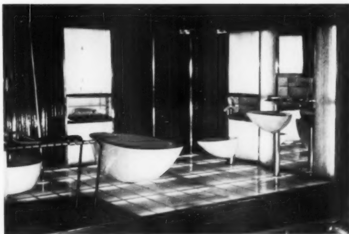
Electronic bathroom (Jules Weydts, Belgium) replaces valves with simple pushbuttons mounted in recessed stainless frame with snap-up front. One button controls temperature of water, which flows into bowl from slits under rim. System operates bathtub by remote control if desired.
