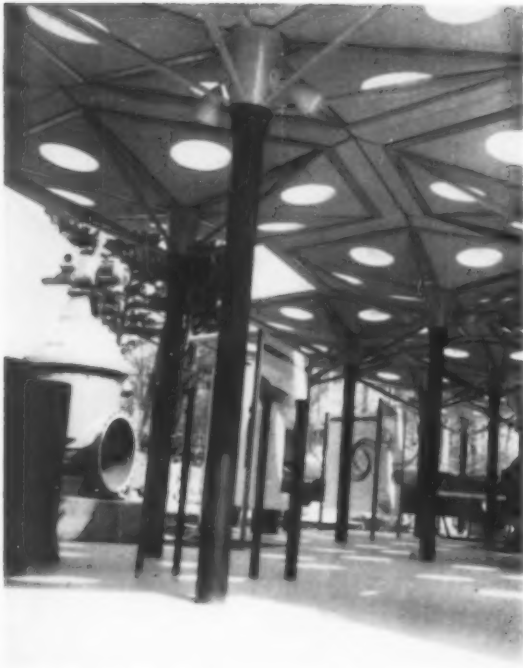
Perforated umbrellas on steel stems form simple open shed for France's Ponts et Chaussées.
