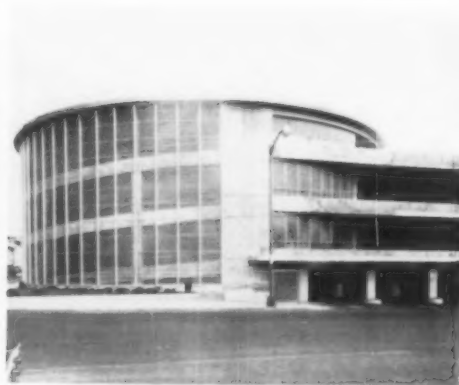
Translucent Buffalo, N. Y. garage wall of shatterproof fiber glass made by Alsynite Company.
