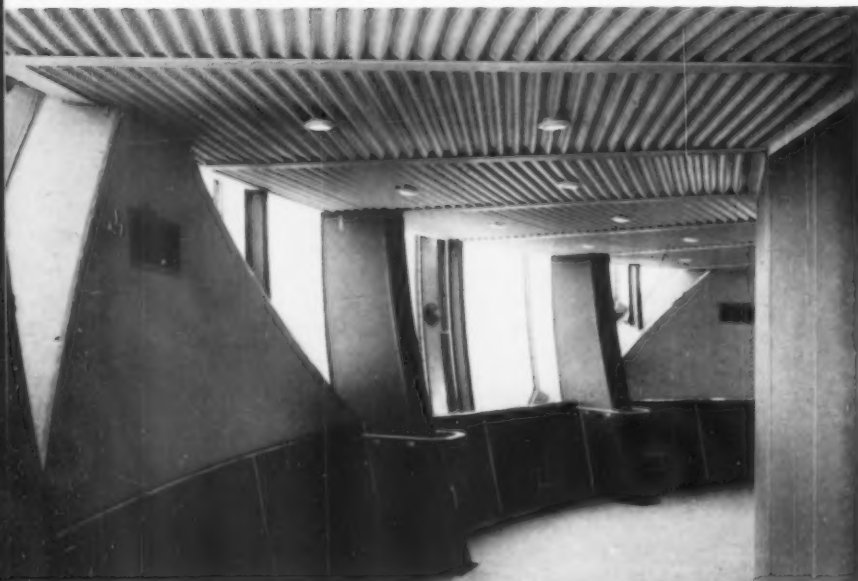
Panoramic outer corridor of Atomium's upper sphere has bulk-head partitions of blue Colovin vinyl in the Munster (linen) pattern laminated to steel. Despite heavy traffic, color and finish have remained fresh with a minimum of maintenance.
