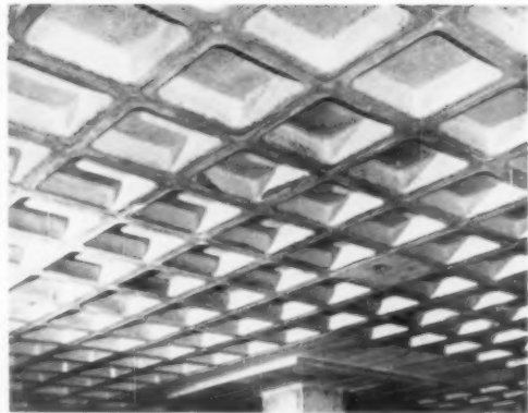
Reinforced plastics forming pans from Protective Plastic, Ltd. were used to form this concrete roof.
