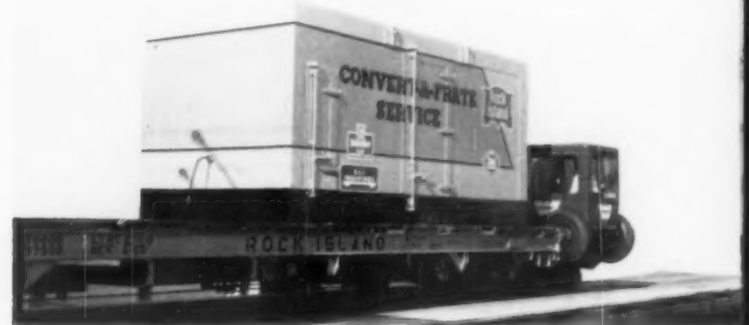
Refrigerated cargo unit Convert-A-Frate was made of reinforced plastic panels assembled as a box car. Made by Minnesota Mining and Manufacturing Company.
