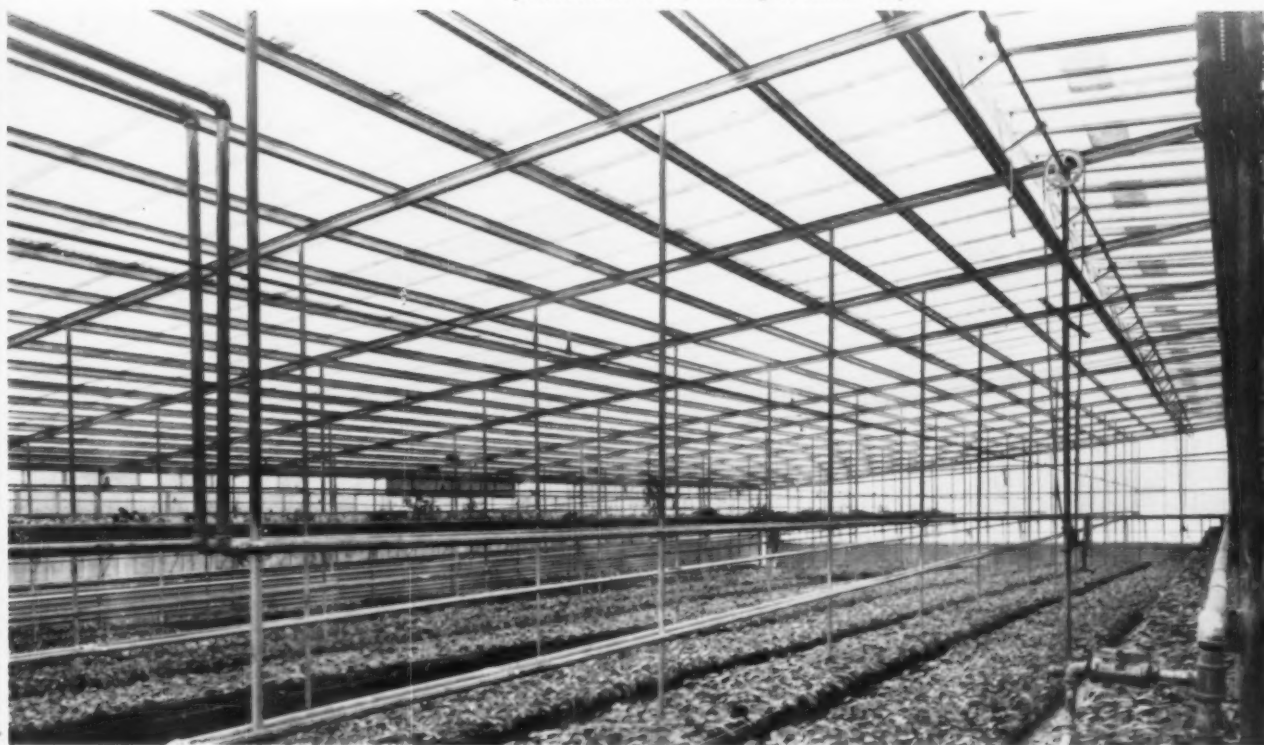
75,000 square feet of fiber glass Alsynite panels clothe this Florida greenhouse roof.
