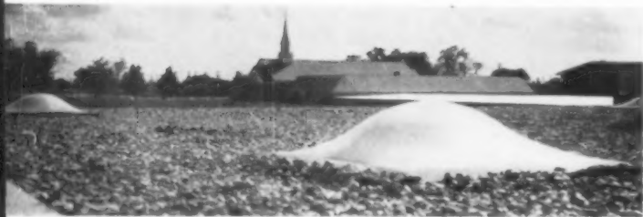
Weatherproof fiber glass skylights made from Celanese Corporation's Marco resin.
