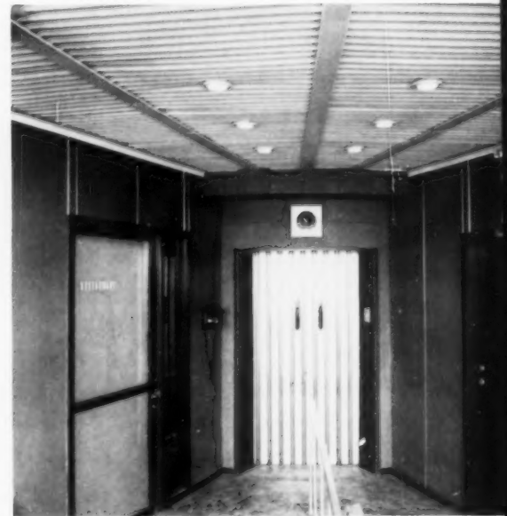
Entrance hall of the Atomium Restaurant, as well as the circular lobby, features a ceiling formed of cream-colored Colovin-on-aluminum panels. The material is perforated and waved to deaden sound. Similar ceiling is used in the corridor at left.
