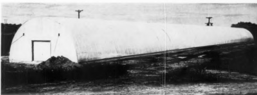
A 340' x 30' giant air-supported building built by the G. T. Schjeldahl Company from polyester resin reinforced by a grid of nylon fibers which prevents tearing.
