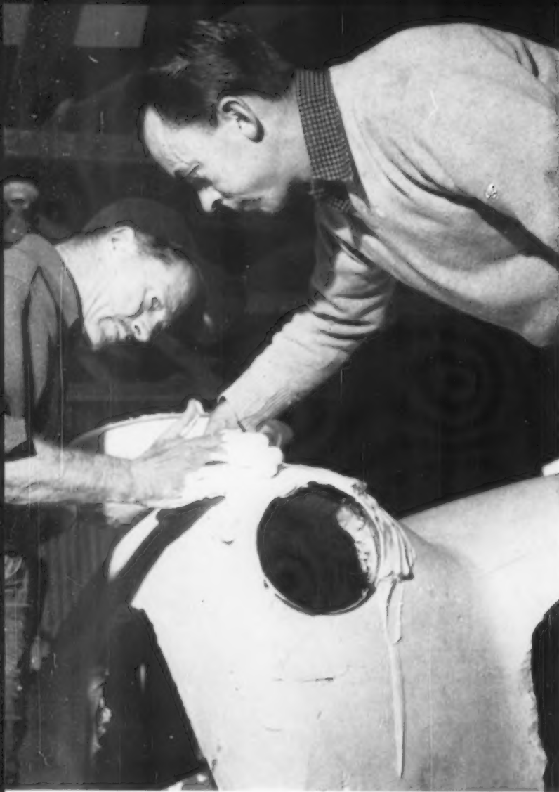
First step in making reinforced plastic body by hand, is shaping the mold. Inexpensive wood and plaster male mold at left served to fabricate experimental car body for joint venture by U.S. Rubber Company and Glasspar Company, in 1952. (Above) roller is used to apply resin to reinforcement built over mold in hand lay-up process.
