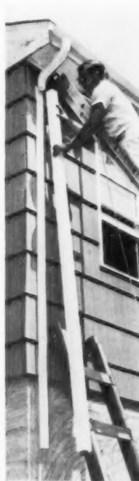
Gutters and drainpipes are a promising new field for reinforced plastics. Those shown are made by Permanent Products, Inc. Owens-Corning is the national distributor.
