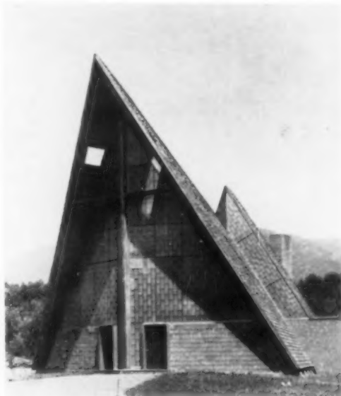
Stained glass effect given front wall of this church by multi-colored sandwich panels from Kalwall Corp.
