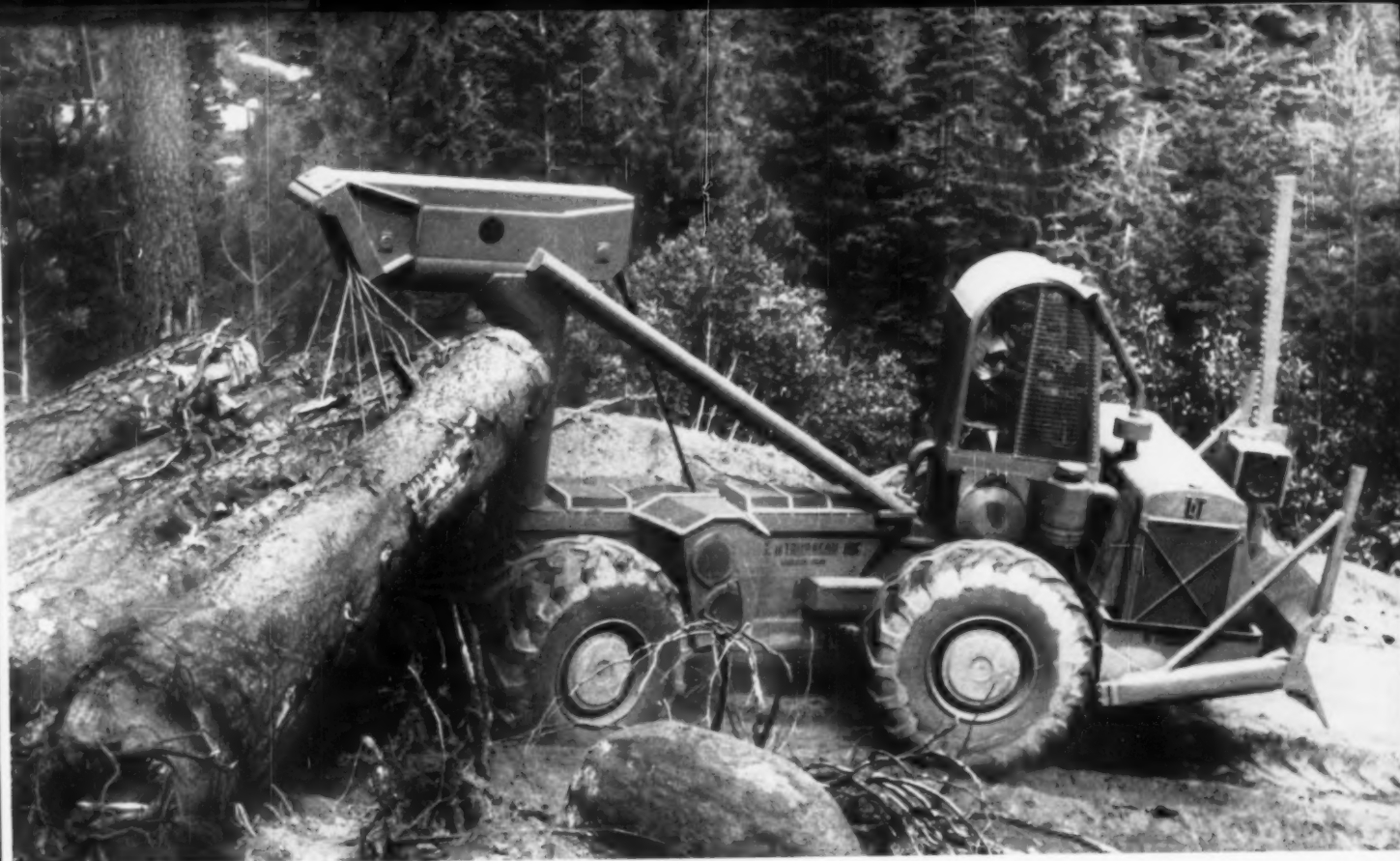
The Log Hauler has been especially designed to move heavy timber over rough, unimproved logging roads. One of a family of LeTourneau logging machines, this mammoth also is powered by electricity.
