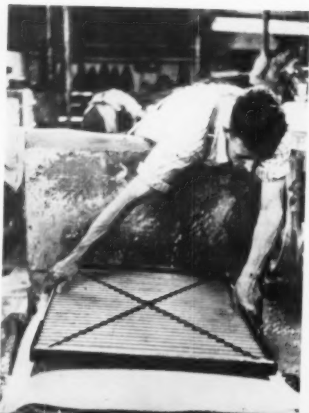
3 Coucher laying newly formed sheet of paper from mold given him by vatman. The mold upside down, the paper is placed between sheets of felt. This is called the "post."
