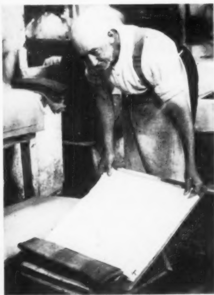
5 The "layman" piles neatly pressed sheet of paper on his inclined table. He removes the felts and returns them to the coucher. Vatman, coucher, layman form "trinity."
