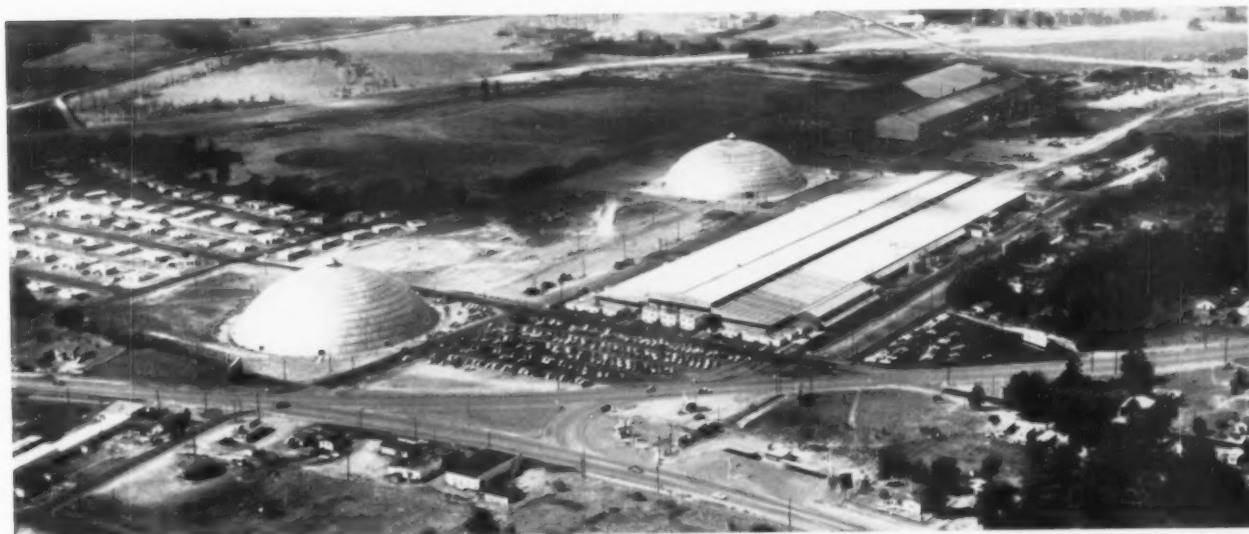
Two huge aluminum Hemispheres dominate the LeTourneau plant at Longview. LeTourneau-designed building stand at the left.
