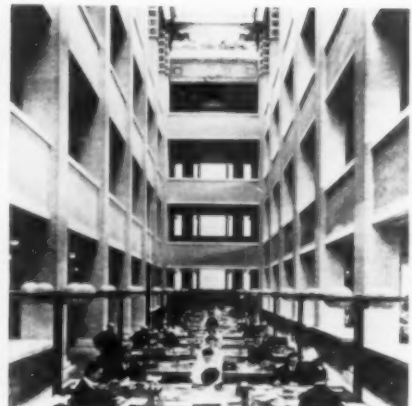
Wright's Larkin Building
