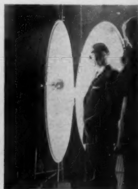
C New, powerful fluorescent-mercury lamp of Westinghouse (right) for street, auditorium and industrial lighting.
