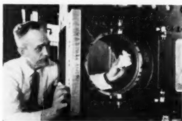
Optical purity and a high softening point (1585° C.) make Corning's 100% Fused Silica useful in wind tunnel windows.
