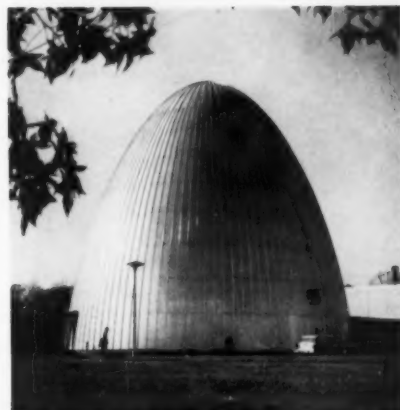
"Beehive" structure is home of reactor. The 87-ft. aluminum dome is center of jointly owned Industrial Research Labs, Inc.
