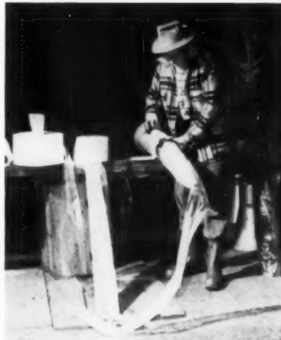
Because of a new packaging technique, fresh Christmas trees may now be shipped to any part of the country, and stored without shedding. Polyethylene sleeve retains the tree's moisture, reduces fire hazard, and cuts shipping space in half. Using funnel-shaped device which guides trees in sleeves, two men can package over 500 trees a day. Designed by E. B. Robbins.
