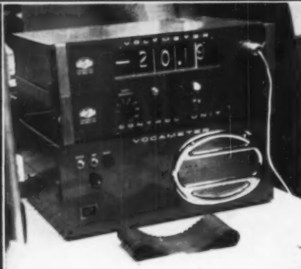
Novelty exhibits at IRE show included a demonstration by Martin Company of man in full pressure suit and proper chair for space flight, and Cubic Corporation's voltmeter with vocameter attachment which "voices" volt readings shown on voltmeter; tape in front of meter (above) stores recorded readings. Emerson & Cuming, Inc. introduced a new dielectric material, Ecospheres (left), made up of hollow glass microspheres, to improve insulating properties of plastics, rubber. One of the largest products shown was shakers and control console (below) by Ling Electronics Inc., which can create powerful vibrations for noise and sine wave vibration testing.
