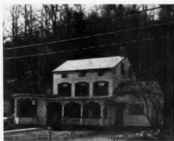
Hudson's main offices are in this 120-year-old house in Croton, N. Y. Other storage facilities and fabricating shops are scattered all over New York's Westchester County.
