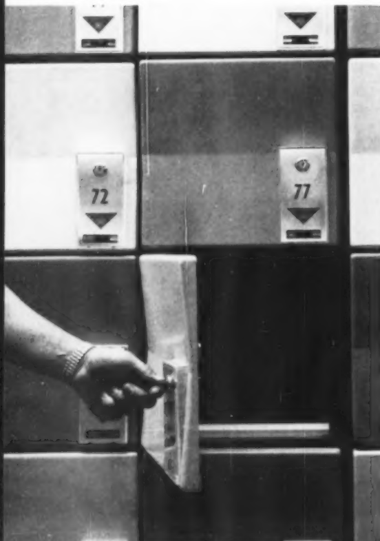
Canted-front lockers have gasket edges to cut down noise; floor is recessed to keep ball from rolling out. Locker's key is its knob, eliminating any protruding hardware.
