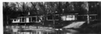
Stubbins' house in Rhode Island.
