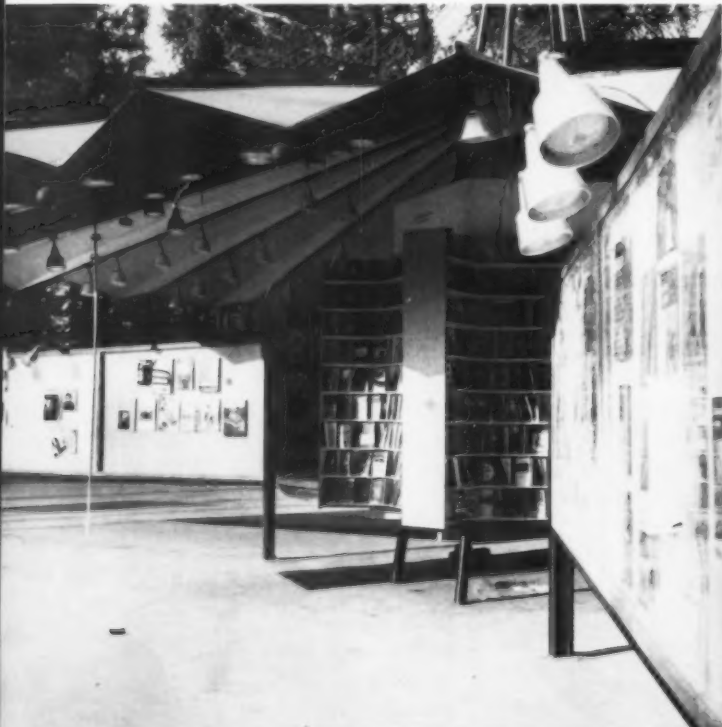
Colorful canvas tents, designed by the Nelson staff, are constructed on umbrella principle—central A-frame supports ribs which open like umbrella when raised to proper height. They covered displays of paperbacks and magazines (tacked on board) and beauty salon, among others.
