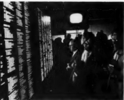
Russians studied 4000 possible questions to put to the RAMAC. Operator fed question to machine. Answer appeared on one of two typewriters and was also flashed on a tv screen for all to see.
