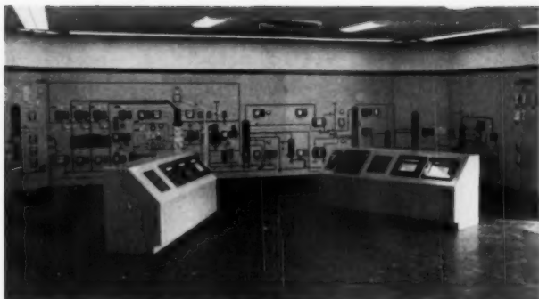
Refineries everywhere are controlled from central systems such as the installation at the Pointe au Tremble, Montreal, refinery of Canadian Petrofina Ltd. Data is read on multipoint recorders in the foreground. Process flow is indicated on panel in the back. System is controlled electronically, transducers are employed to convert force into dc signal. (Manning, Maxwell & Moore, Inc.)
