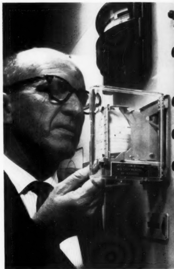
Pneumatic tube transmission is being adapted to automatic operation by combining it with modern control devices. All inter-office communication at Standard-Vacuum Oil Co. in White Plains (N. Y.) is taken care of by automatic tube carriers (right). Movement is recorded by lights on control panel. (System by Airmatic Systems Corp.).
