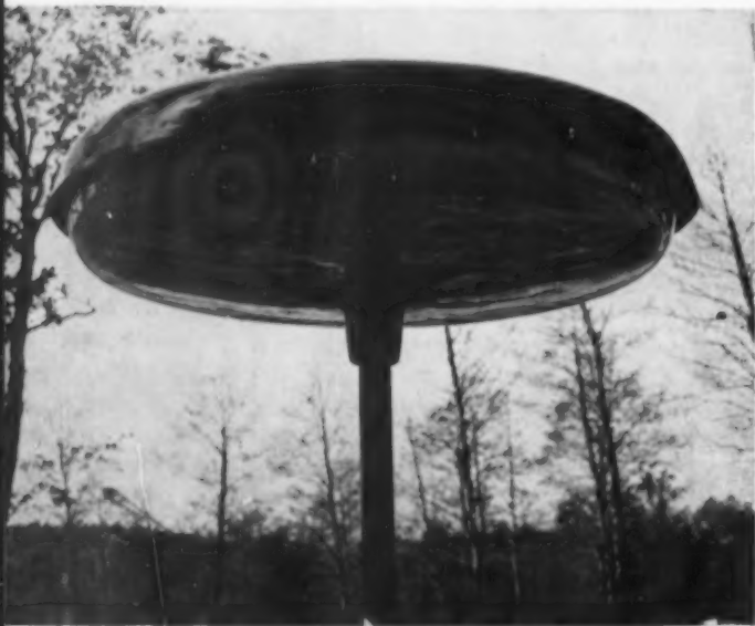
Post top fluorescent lantern with polyester canopy and acrylic plastic bowl. Designed by Per Heribertson.
