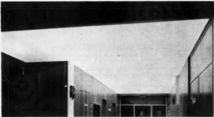
295 Luminous ceiling Integrated Ceilings, Inc., Los Angeles Staff design
