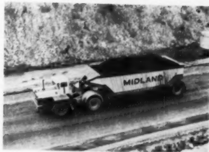
263 Coal hauler LeTourneau-Westinghouse Co., Peoria, Ill. Box-beam-and-corrugated trailer construction of high-tensile-strength steel; air-actuated bottom-dump doors.
