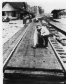
249 Rubber track cushions Goodyear Tire & Rubber Company, Akron Rubber railroad crossings for motorists over a double set of curved tracks at Wooster, Ohio; eliminates ice collecting, bumps.
