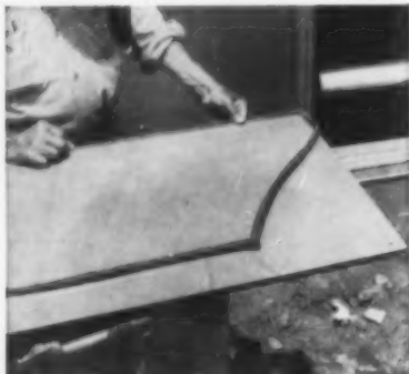
Easily installed — Butyl preformed gaskets can be installed on-site or in the shop. They protect panel edges during handling.
