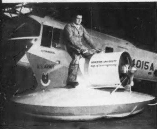
245 Air Scooter Princeton Department of Aeronautical Engineering, Princeton University, Princeton, N. J. Not strictly a land vehicle, scooter resembling a Flying Saucer rides at a height of 3 to 4 inches above ground; is 8 feet in diameter at base.
