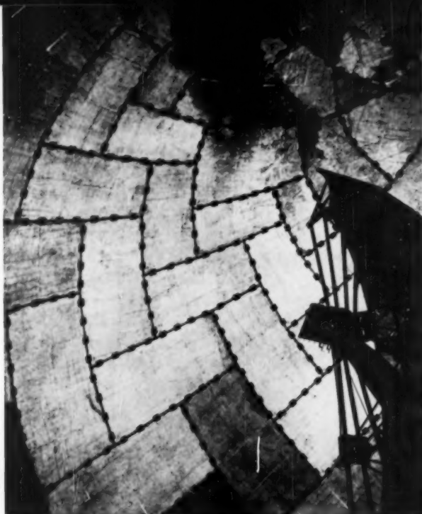
These fasteners used to join radome fiberglass panels also contribute pattern; Simmons' DUAL-LOCK.
