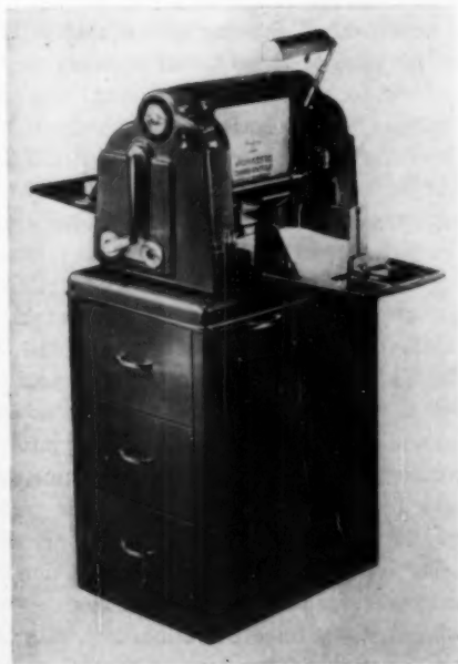
1953 Model 260 expanded automation: inking was fully automatic, and so was copy-counting.
