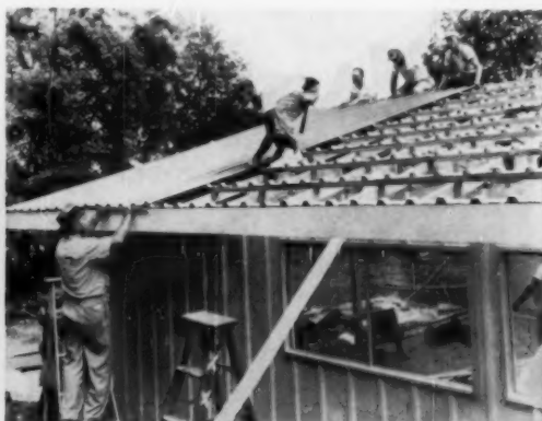
Pre-assembled structural panels of Viking house are erected on site (left), then aluminum siding is laid over them. Roof panels (center) fit over pre-formed aluminum hangers. National, which also makes wood prefabs, offers the Viking Line in numerous models, among them the Fair-L-Wood (right) in California Contemporary style, designed by Charles Goodman.
