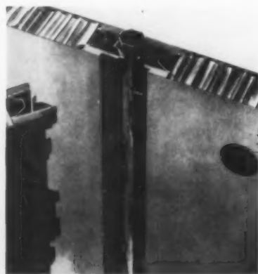
Joining system for paper-cored aluminum panels, designed at IIT, uses brackets that clamp around octagonal post.
