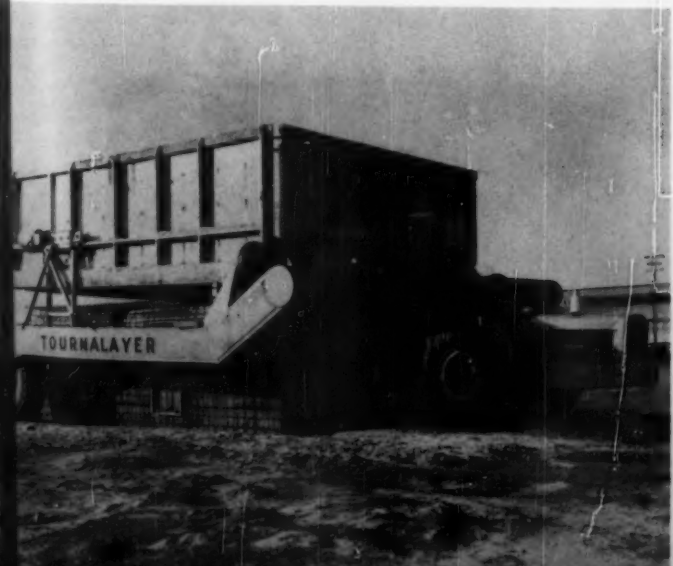
9. Le Tourneau's cast-on-site concrete house
