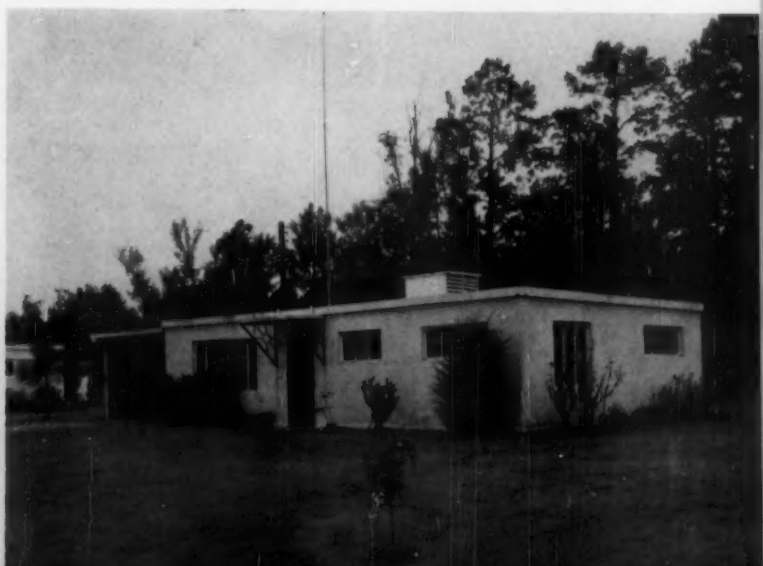
9. Le Tourneau's cast-on-site concrete house
