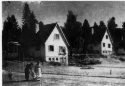
In Finland (two photos above) prefabricated houses are made entirely of wood, using traditional structural systems; many do not even use plywood. Design is prosaic, but carpentry is excellent.
