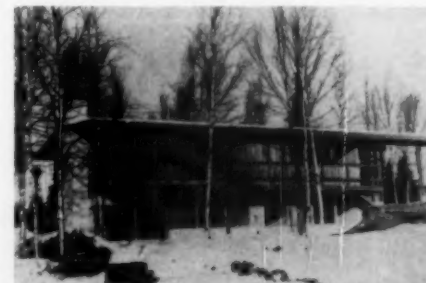
Two other examples of U. S. prefab operations are Loetwall Corp. whose houses (top) are assembled from stressed-skin plywood structural panels, and Modular Homes (below) which uses post-and-beam construction, modular curtain wall panels.
