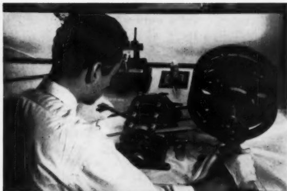
Henry Trettin runs off rushes in PGL cutting room while Anthony J. Ciccolini (foreground) operates Moviola, editing device that runs film at standard projection rate of 24 frames per second, enables editor to determine exact frames at which to cut.
